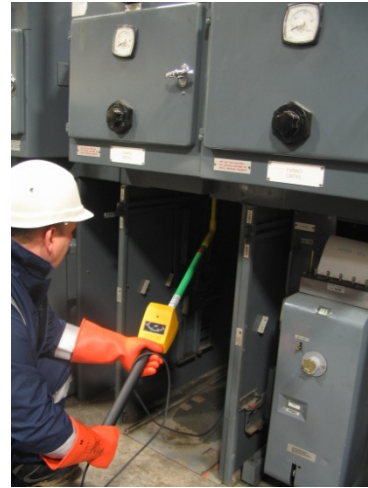
Switchgear Testing
