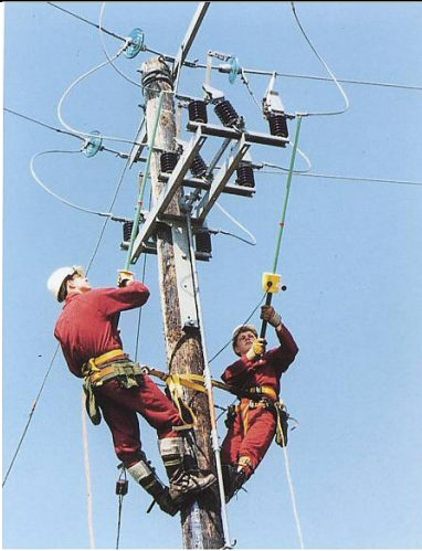
Overhead Line Testing
