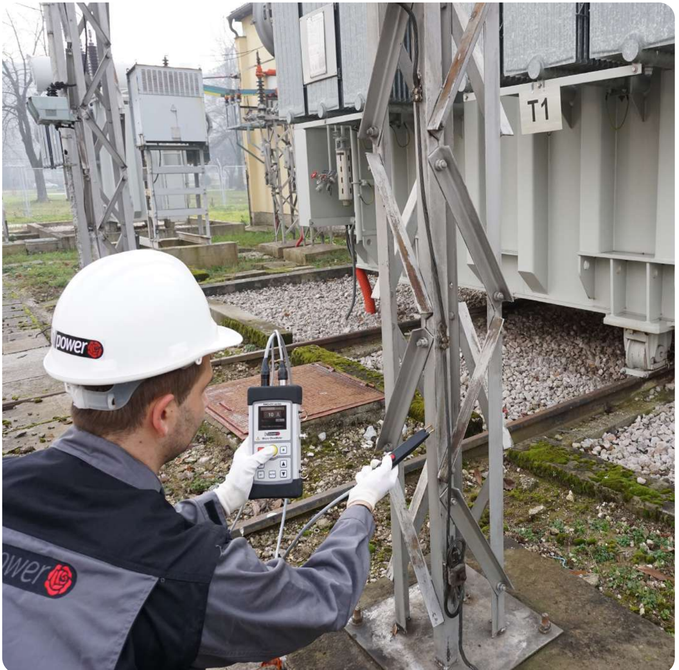
Ground Grid Integrity Test using RMO-EH
